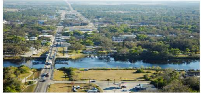
Today’s Riverfront at LaBelle. Existing bridge is to the left. The proposed FDOT second bridge and its off-ramps, embankments, ETC. would be built in the small space between the City Docks and the Barron Library (center of photo) and the existing bridge.
